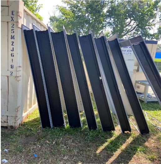
Hollow Metal Frame Damp Proofing
