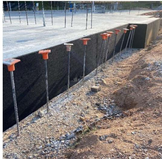
Slab On Grade Expansion Joint
